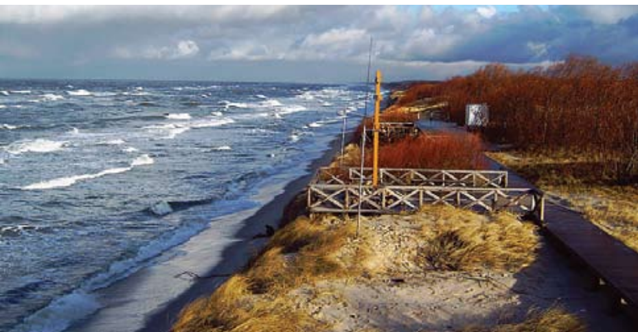
Fig. 20 b. The extensive washed-out locations (up to 8 m in width) appeared along the pipeline
