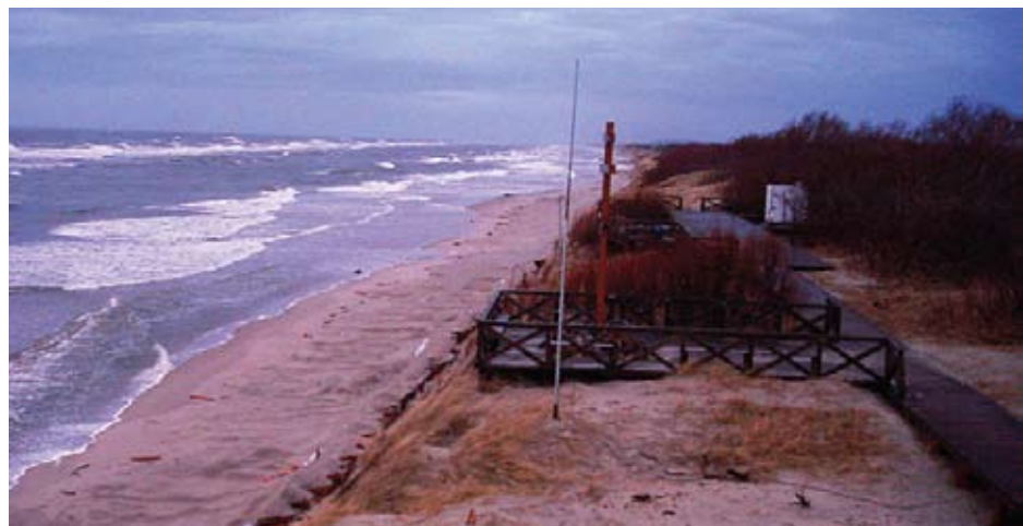
Fig. 20 a. The extensive washed-out location (215 m) near the pipeline outlet to the bottom surface
