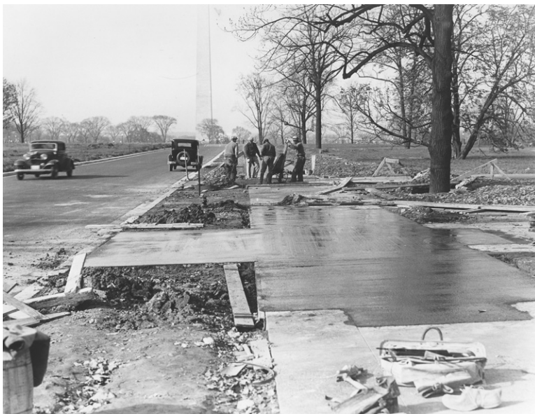
In 1935, concrete sidewalks were built along the outer edges of the Mall Vista Drives. (from MRCE; CLP file "Mall laying sidewalk 1935")
