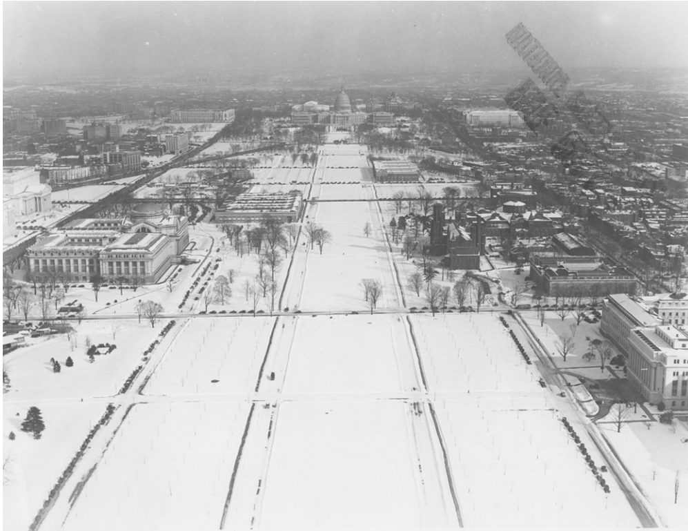
By 1936, the power plant had finally been removed. This photograph was probably taken early in the year. (from MRCE; CLP file "Mall from Wash Mon 1936")
