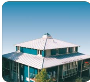
EN 1.4510/430Ti (standing seam technique), Ugine & Alz, 독일
