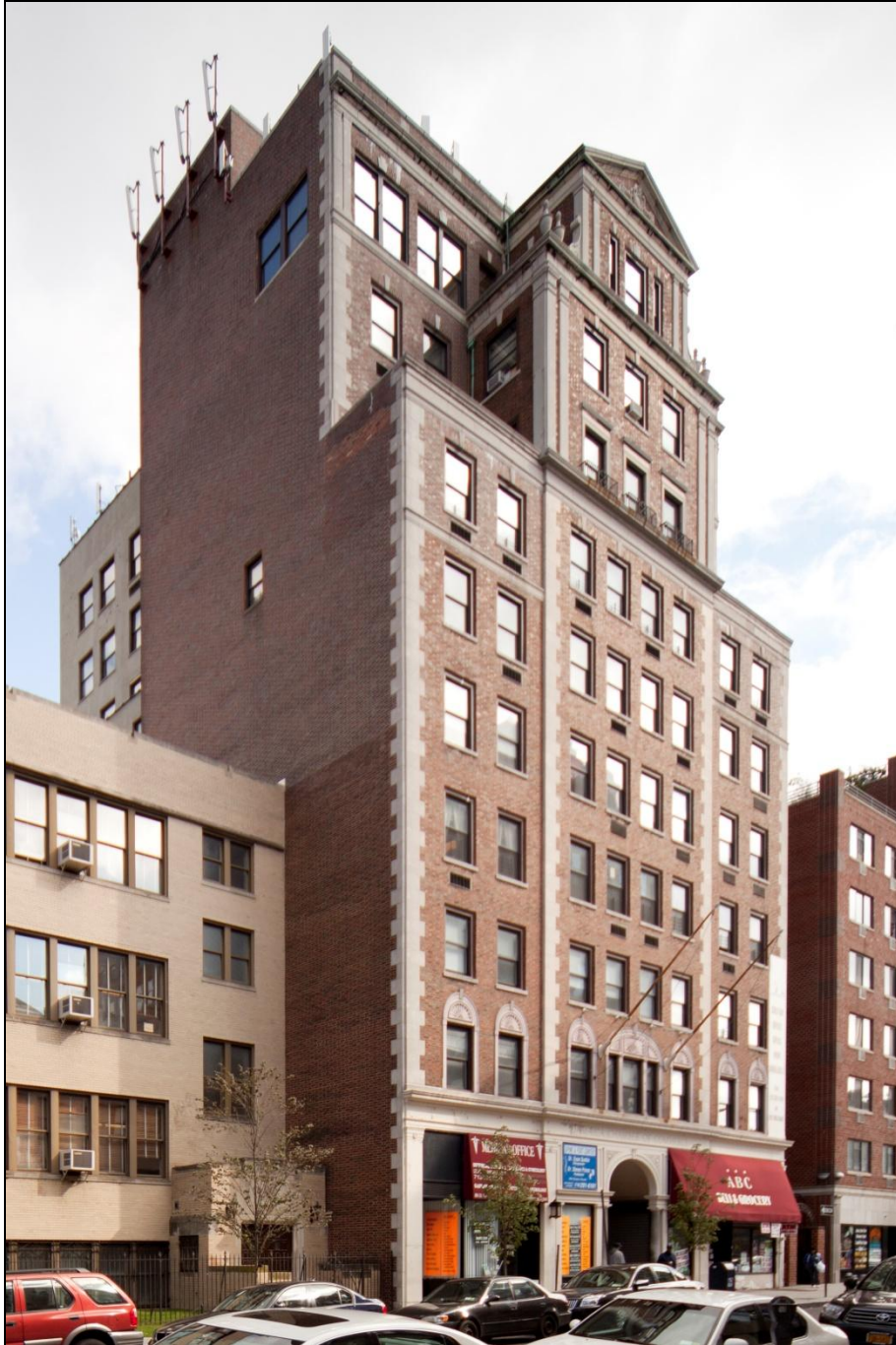
Jamaica Chamber of Commerce Building View from the northwest Photo: Christopher D. Brazee, 2010
