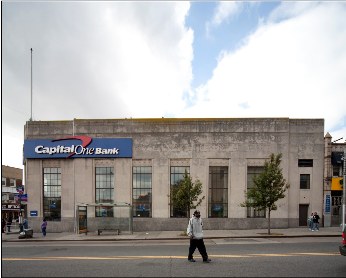
Jamaica Savings Bank Sutphin Boulevard facade Photo: Christopher D. Brazee, 2010
