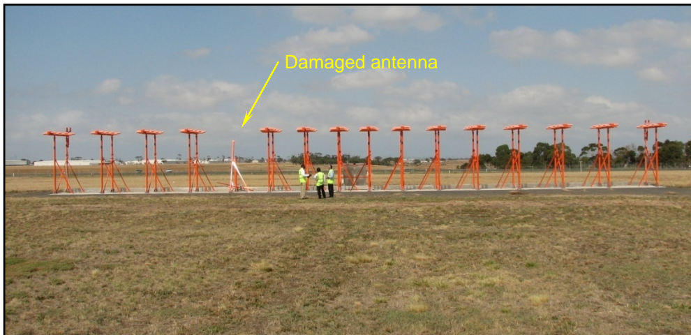
Figure 12: Localiser antenna array
