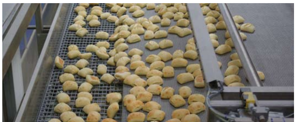
Final baking of the partly-baked bread rolls. The entire conveying technique has been installed by Kaak.
