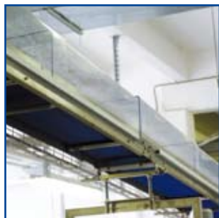
All conveyor belts are protected by a transparent plastic cover in order to avoid any influence of the room climate on the dough pieces.
