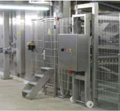
The hearths in the Automatic Hanseat at Lantmännen are divided into a pre-baking and a final baking zone.
