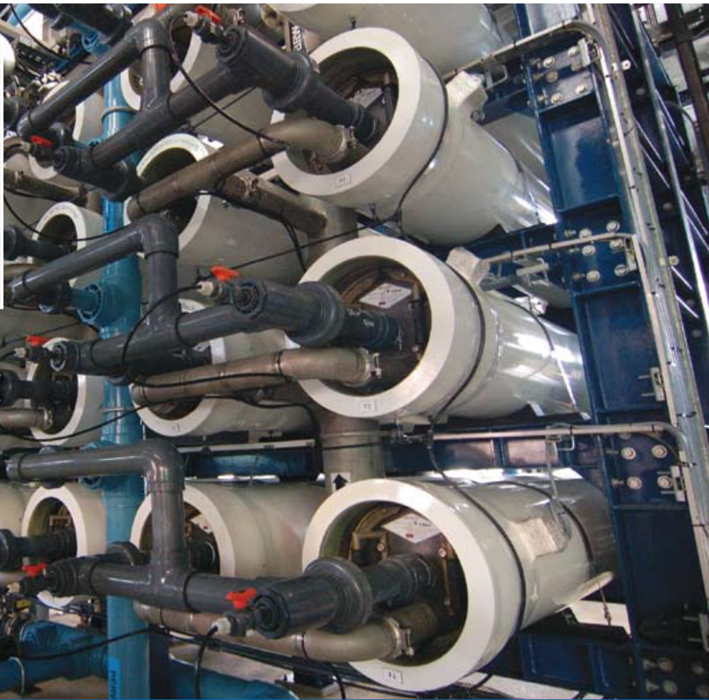
CH2M HILL Project Manager Ho Chee Yon and Commissioning Engineer Felix Wang (above) conclude performance tests at PowerSeraya's new SWRO plant, the world's first full-scale SWRO plant with 16-in. diameter pressure vessels.
