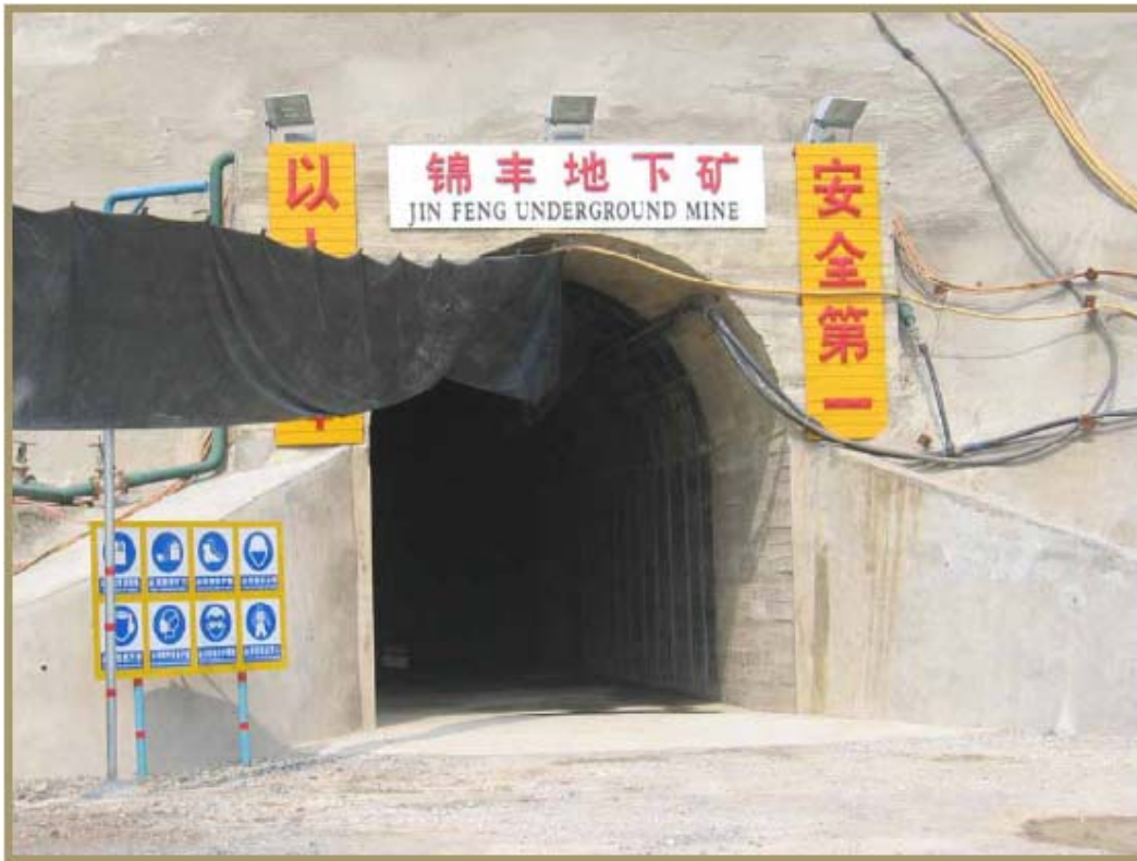
Figure 5-1: Jinfeng underground mine portal
