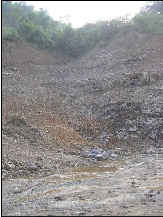
Figure 17-23: CIL Embankment Construction, 15 October 2006
