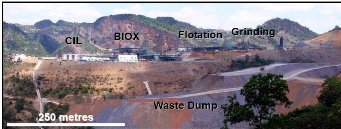
Figure 17-25: Photograph Showing General Plant Layout, April 2007
