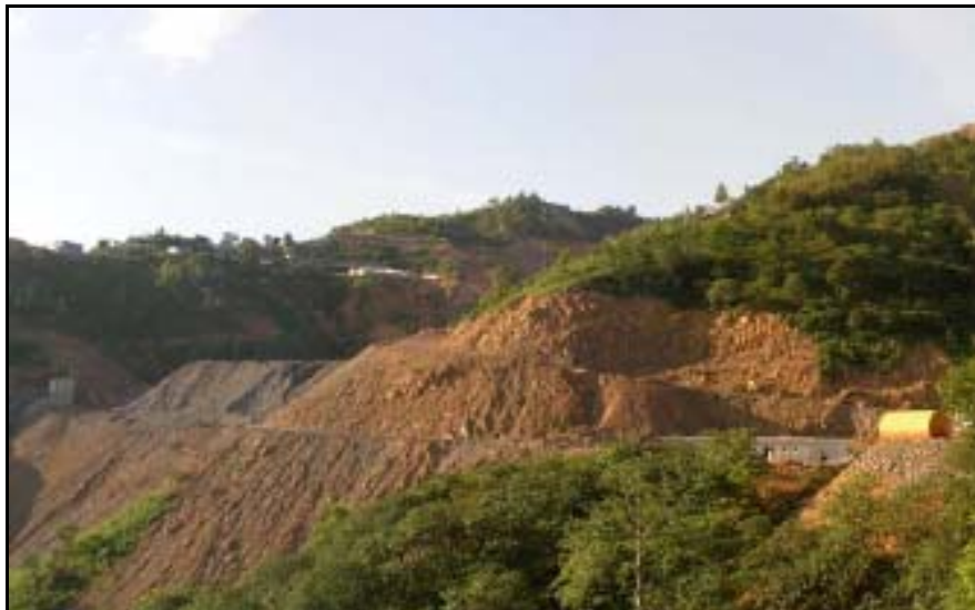
Figure 17-6: Photograph Showing Main Decline Portal Area, 15 October 2006
