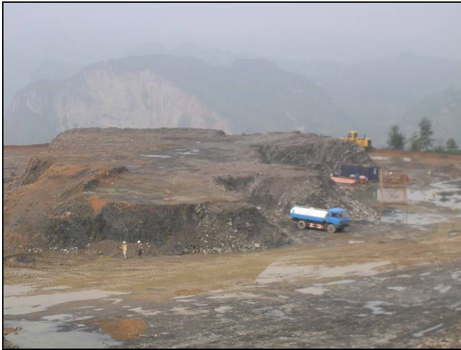
Figure 17-2: Photograph Showing Open Pit as at 15 October 2006
