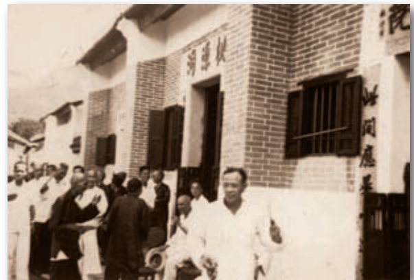
A building complex in Wun Yiu's To Yuen Tung. Longevity Chamber is on the right. Many devotees visit To Yuen Tung during its festival. (Provided by To Yuen Tung)
