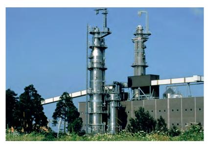
2205 continuous sulphate pulp digester and impregnation tower, Sodra Cell Mönsteras, Sweden (Source: Kvaerner Pulping)
