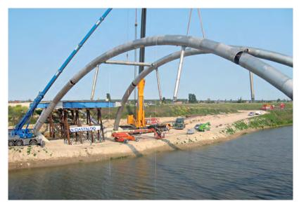
2304 duplex stainless steel bridge arches in construction near Padova, Italy (Source: ArcelorMittal)
