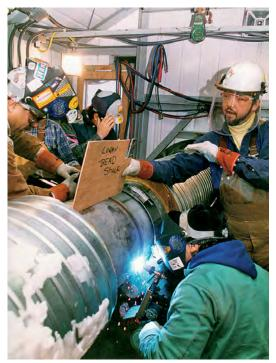
Mechanized welding of large diameter duplex stainless steel cross-country pipeline (Source: Arco Exploration and Production Technology)
