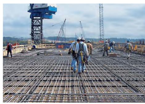
Installation of duplex stainless steel rebar on a large bridge deck (Source: Hardesty & Hanover, LLP)
