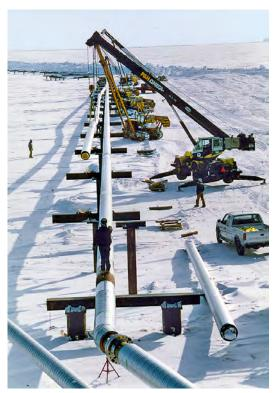
Installation of insulated 24 inch 2205 pipe on vertical support members in Prudhoe Bay (Source: Arco Exploration and Production Technology)
