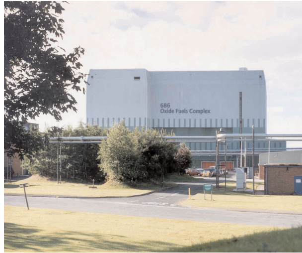
Oxide Fuels Complex, Springfields Site is one of the most advanced nuclear fuel manufacturing plants in the world.
