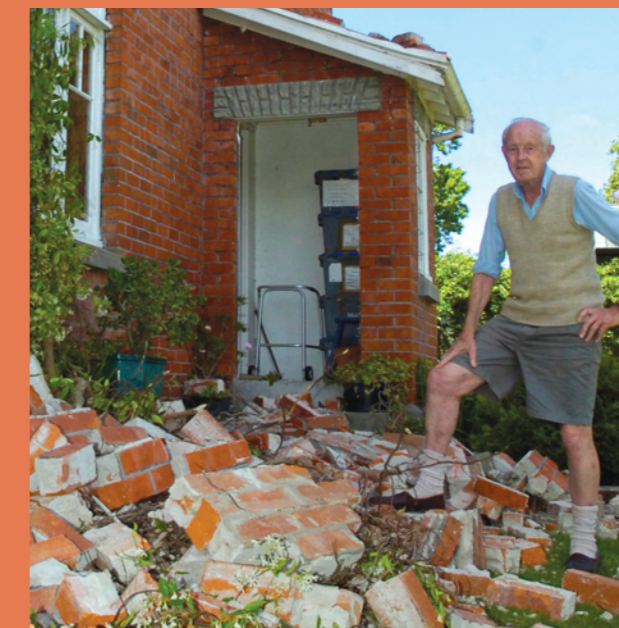
Harold Williams stands among the fallen bricks from the west wall of his house in Gisborne after the magnitude 6.8 earthquake in December.
