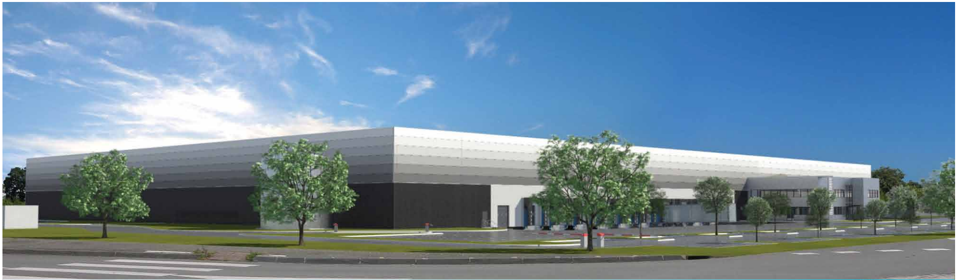
Artists' impression of upcoming Stanley Black and Decker facility in Dole, France
