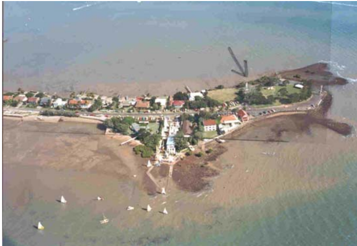
HP1749: the arrow on this photo points to where the Lighthouse is now. It was moved there in 1976. The photo was taken about 1995. Courtesy of Redland Shire Council.
