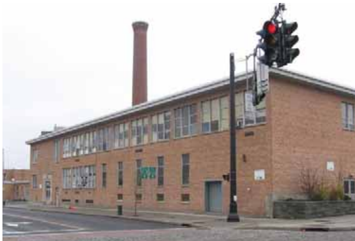
The Rensselaer Street side of Giffen School.
