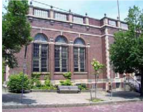
Howe Library on Schuyler Street (between Broad and Clinton) will soon be renovated and expanded.
