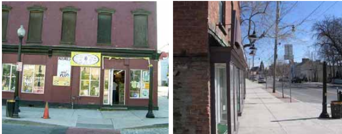
Storefronts along South Pearl Street.
