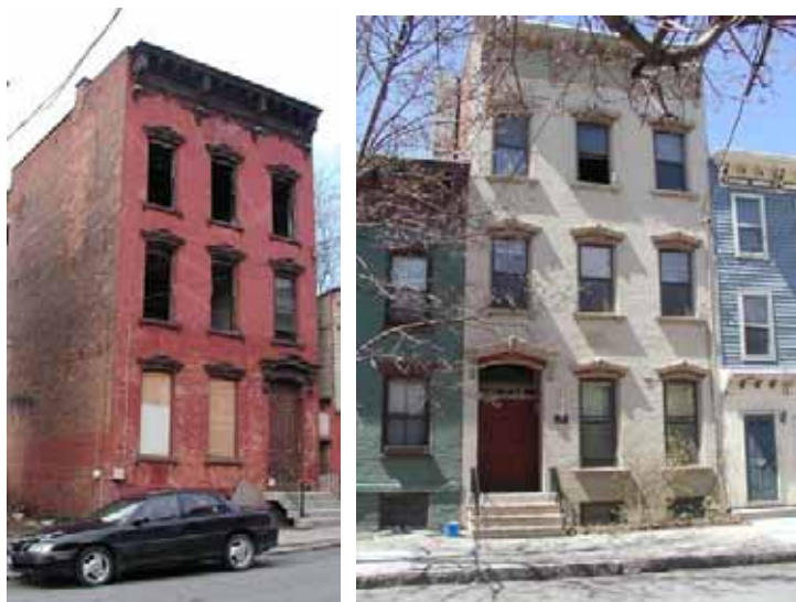
Three story residences: before and after rehabilitation.
