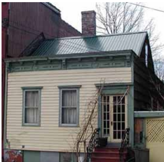
A typical residence, rehabilitated by homeowners.
