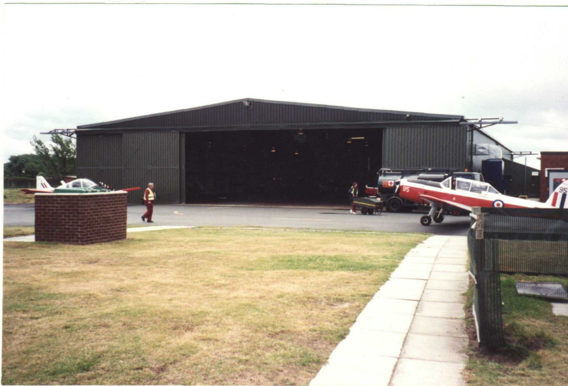
Photo 3.2 External View of Bellman Hangar
