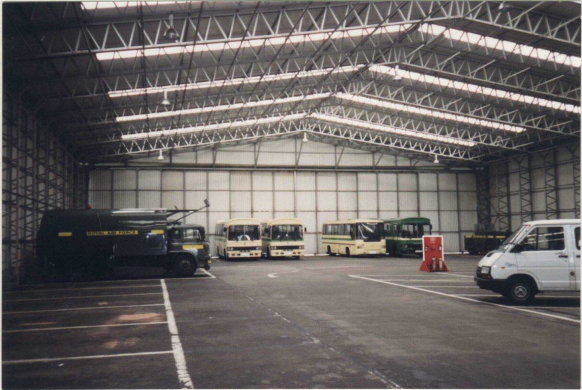
Photo 3.3 Lattice Portal Frame of Type T2 Hangar
