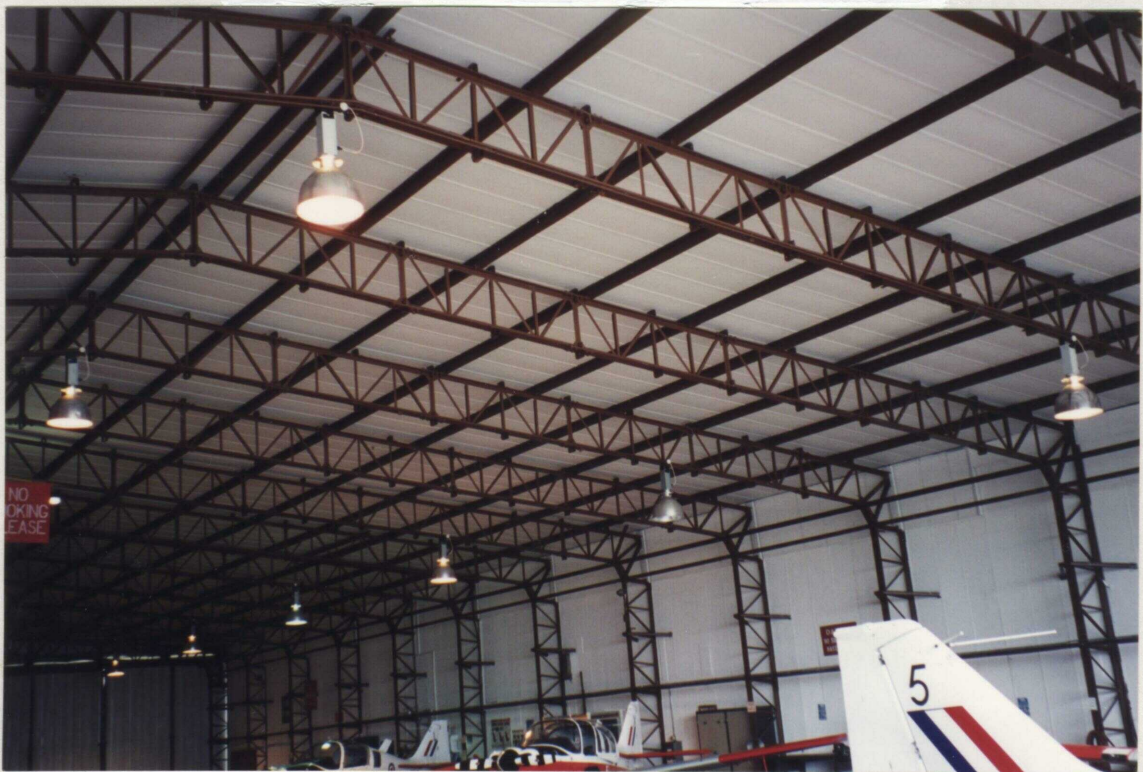
Photo 3.4 Lattice Portal Frame of Bellman Hangar
