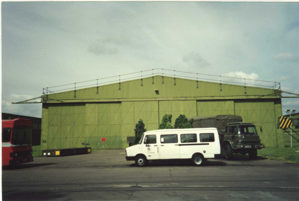
Photo 3.1 External View of Type T2 Hangar
