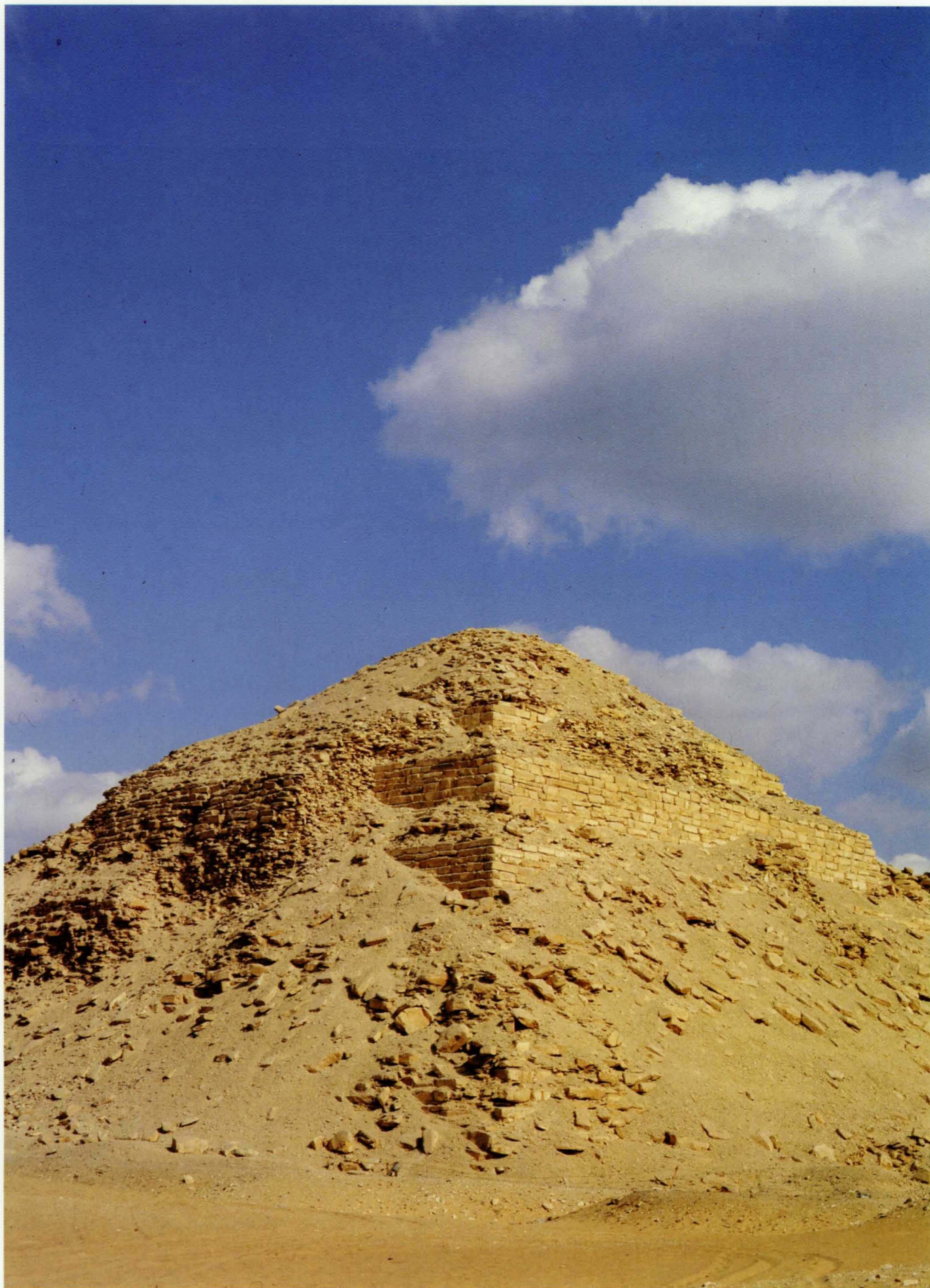
A view of Neferirkare's pyramid from the south west eloquently illustrates the building phases that went into the monument's construction.
