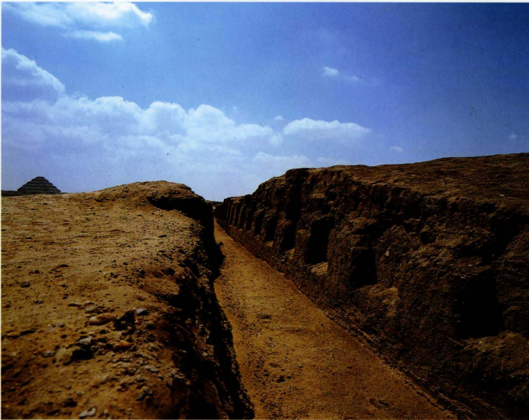
Remains of the facade of the mastaba of Ity (?), Administrator of Both Granaries. 3rd Dynasty. South Abusir.
