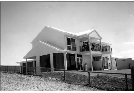
All Aluminum Windows used on this home were fabricated using heavy duty commercial grade Aluminum and custom design french doors. Grey Laminated Safety Glass was used for Security and Performance. The final result looks fantastic!
