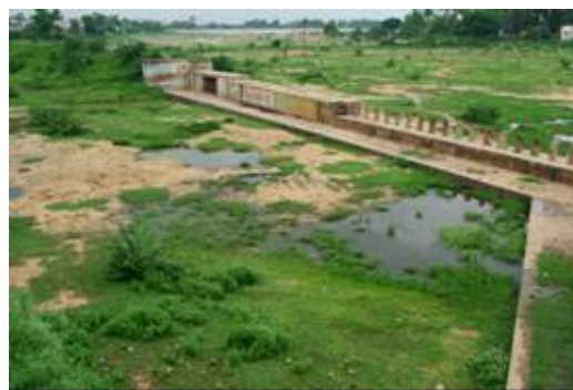
Fig 4.6: View of Periyakulam Kanmoi
