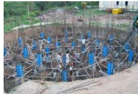
Fig 4.4: Constr. of new OHT at Municipal Office
