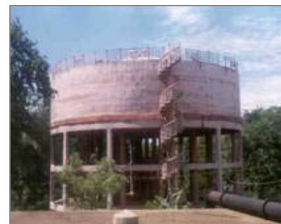
Fig 4.3: View of Kottapatti OHT
