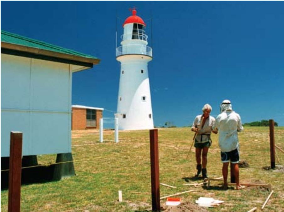
TOP LEFT TO RIGHT: Damage by vandals in lightkeeper's cottage at Bustard Head; Stuart works on repairs at the property; interior of Bustard Head lighthouse. All photos by Stuart Buchanan except interior of lighthouse, which is courtesy of Peter Marquis-Kyle.
