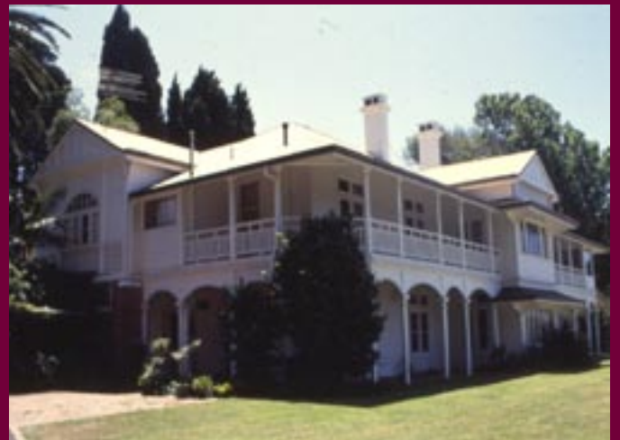
ABOVE: Glen Alpine's grand two-storey verandah.
