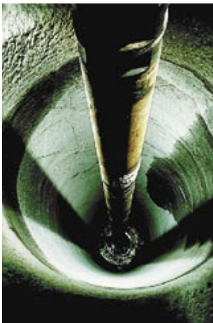
Drilling of a canister hole.
