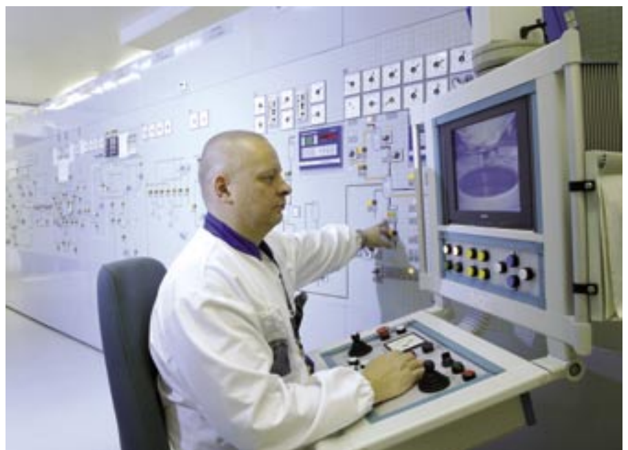
All waste is classified by radioactivity as 'clean', low-level and intermediate-level radioactive waste, decommissioning waste and highly radioactive spent fuel. Waste containing no radioactive substances is classified as 'clean'. It is recycled and the portion that cannot be recovered is taken to TVO's own landfill. Low-level and intermediate-level waste is packed into containers in the power plants.
