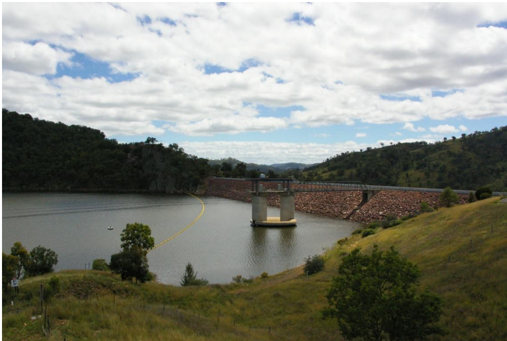
Figure 18: Chaffey Dam spillway.
