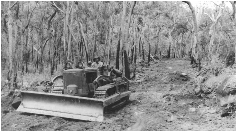
Construction of the 2nd Mount Spec Pipeline 1967
