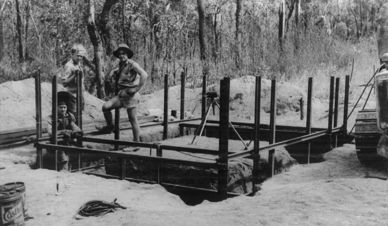
Construction of Mount Spec Pipeline (1958-59)
