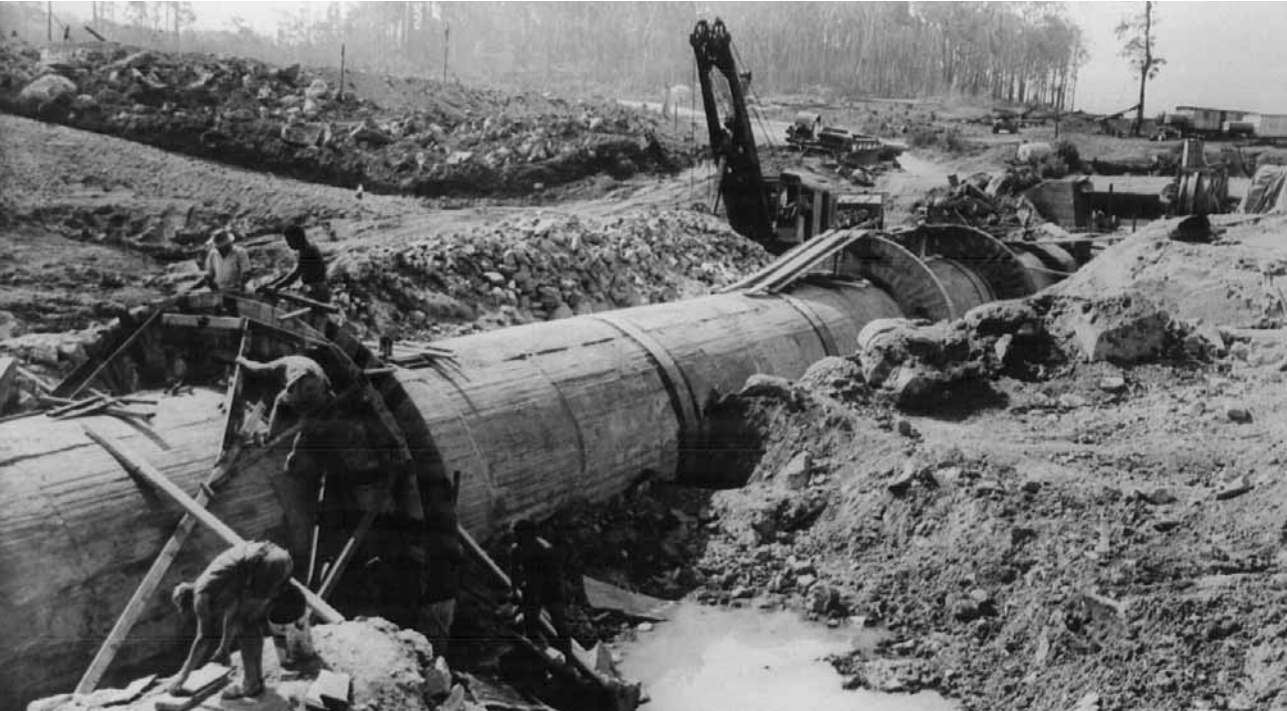
Construction of Paluma Dam 1957
