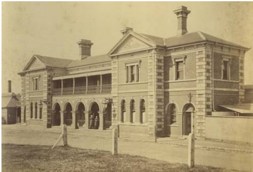
Figure 5.3 Toowoomba Railway Station c1882 (John Oxley Library APO004-0001-0001)
