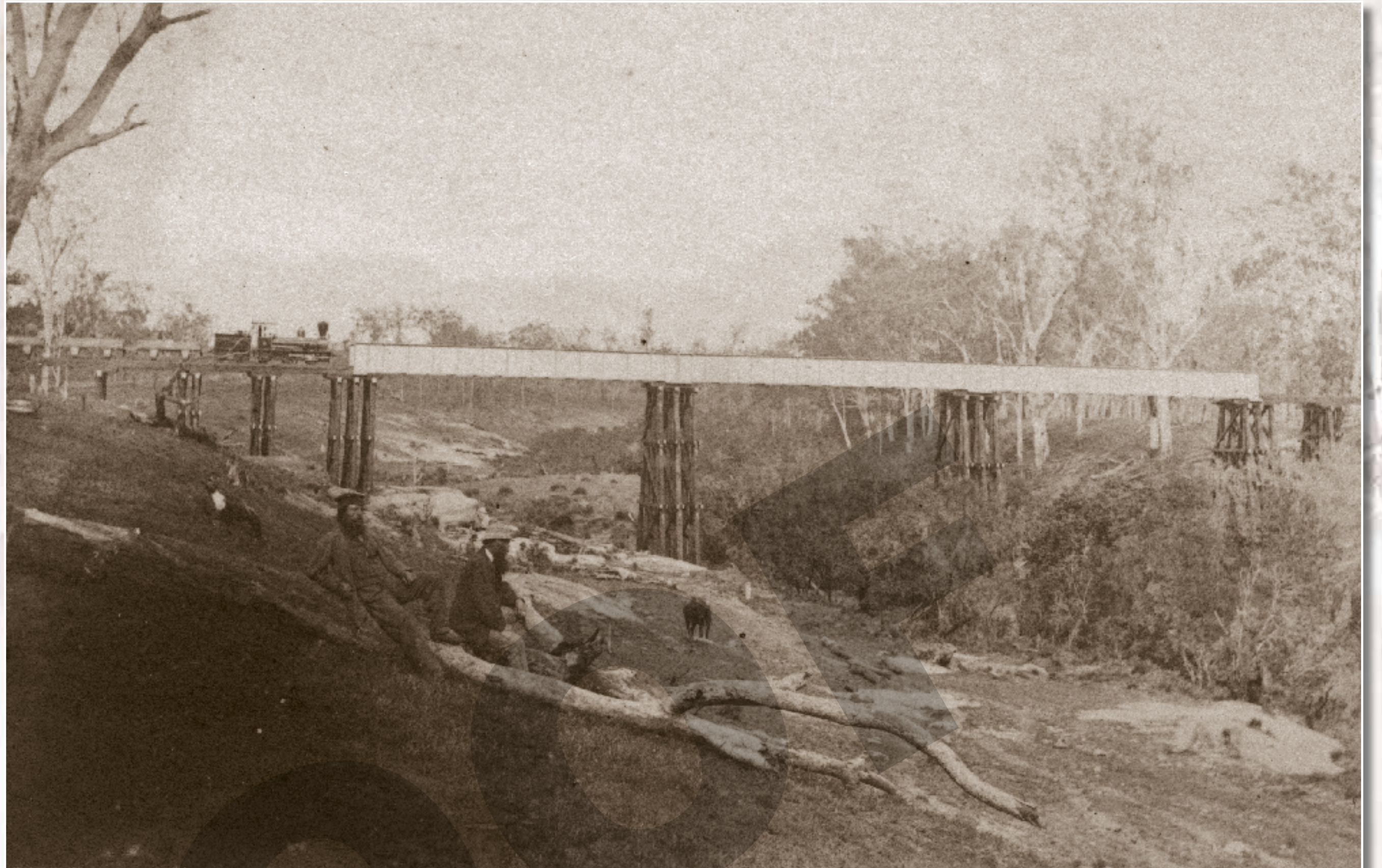
Photograph taken in 1867 at Lockyer Creek crossing at Gatton, showing construction train, and plate girder bridge.
