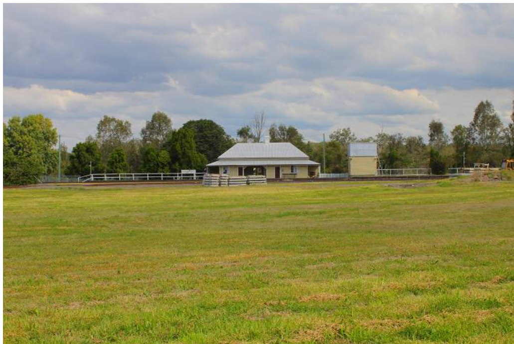
Figure 3.3 View to Grandchester Railway Station from Ipswich Road (ERM 2010)
