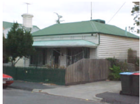
Figure 5 Double-fronted house at No 25
