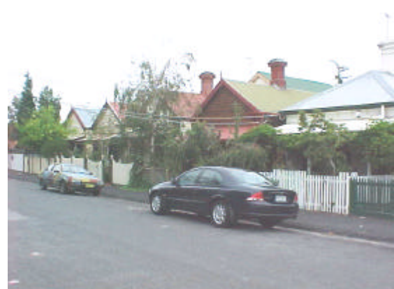
Figure 3 Chusan Street, looking south
