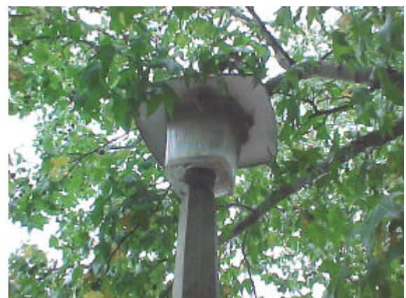
Figure 5 Detail of 1920s concrete lamp
