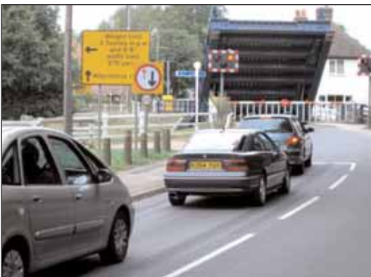
The Lifting Bridge over the canal complete with queuing traffic
