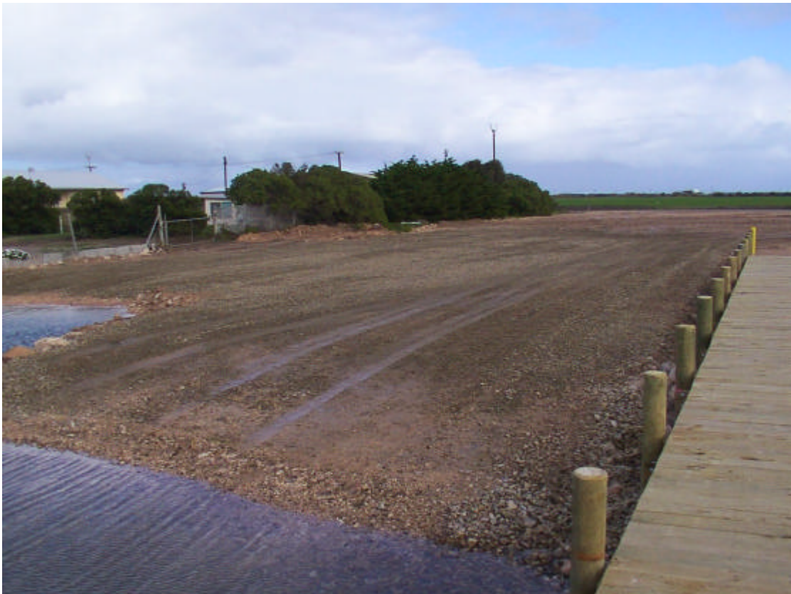
Completed Boat Ramp – December 2003
