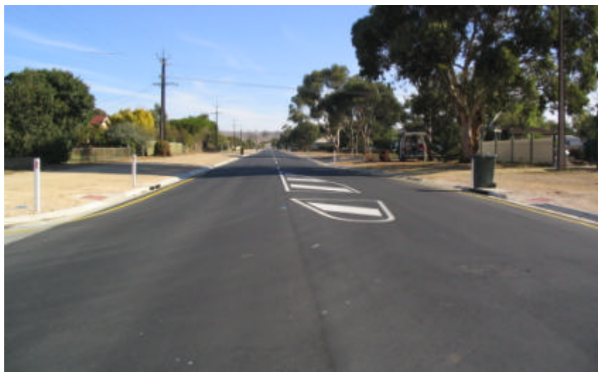
Ashbourne Road Constructed
