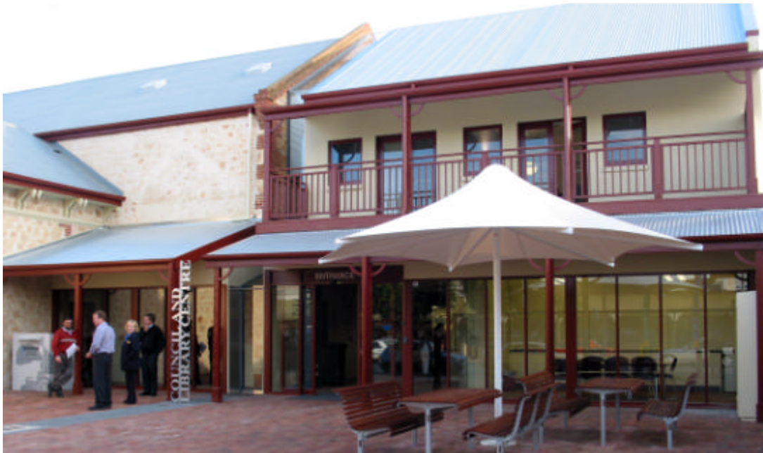
Alexandrina Council Library & Administration Centre
