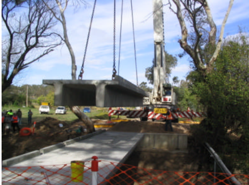
Installation of deck on Kirkham Rd Bridge May 2004
