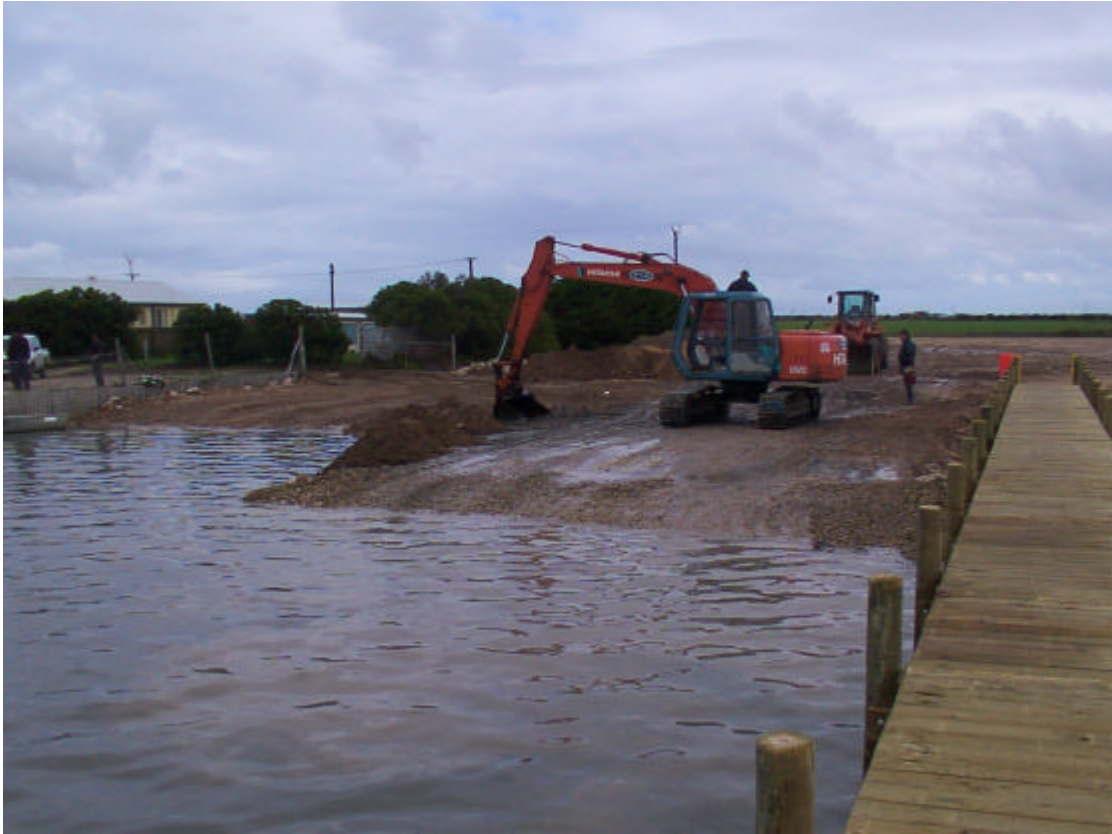
Work being undertaken on Mundoo Channel Boat Ramp
