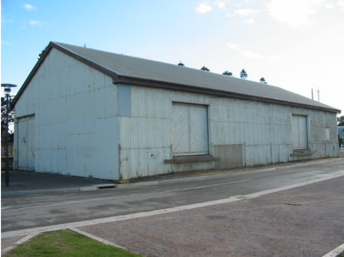
Shed at Goolwa Wharf
