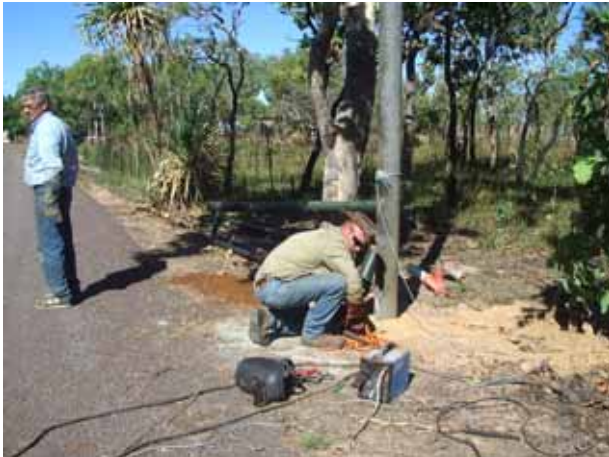
Trevor and Darren working to install the gates running off Dorat Road.
