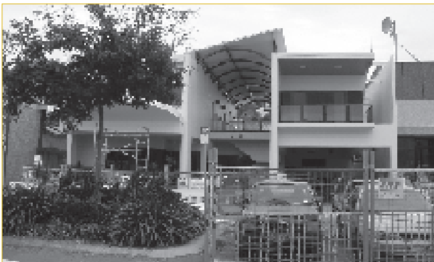
Construction of the new Iris Clay Hostel in Townsville, Qld is under way and it is due to be officially opened in November 2005
