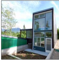
MALONE-DECLAIRE STUDIO , MARBLEMOUNT, WA UNDER CONSTRUCTION, 2008-PRESENT
