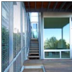
STAIR HOUSE , SEATTLE, WA UNDER CONSTRUCTION, 2008-PRESENT
