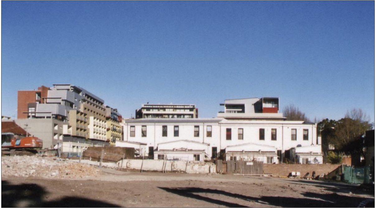
Fig. 12.7 The development site to the north of the temple and the rear of the terrace houses within the temple grounds. The Hudson development towers over the temple to the left and to the south. (Photo: Melita Rogowsky 2004.)
