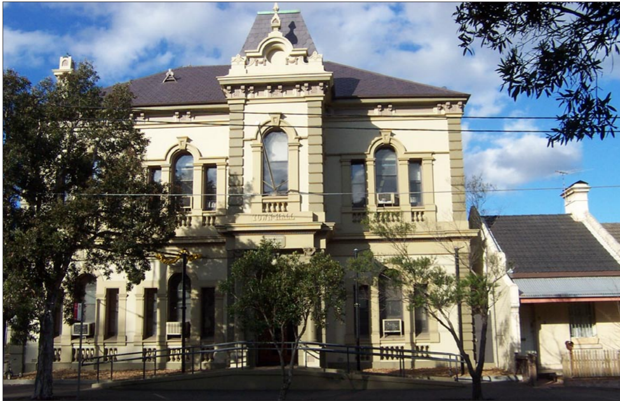
Fig. 8.4 Waterloo Town Hall (now Waterloo Library) where John Charles Hodder was killed in 1965 (Photo: Scott Vance, 2004)
