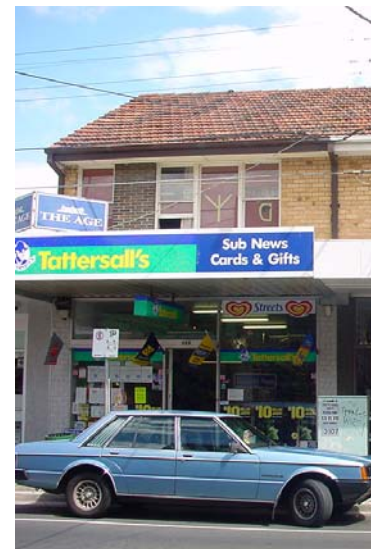
Existing Shop Top forms
