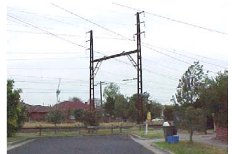
Railway Line Barrier
