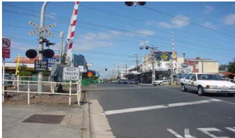
Highett Road Level Crossing
