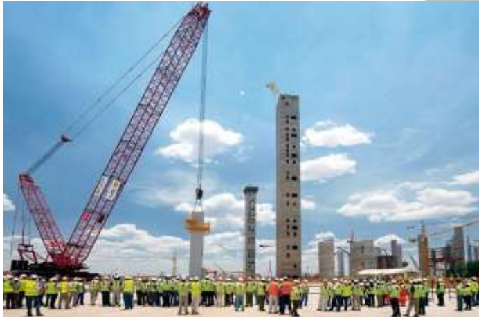
State of construction at Medupi
