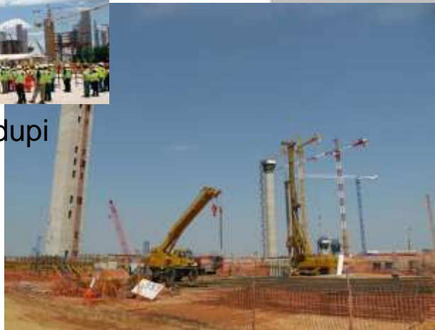
State of construction at Kusile
