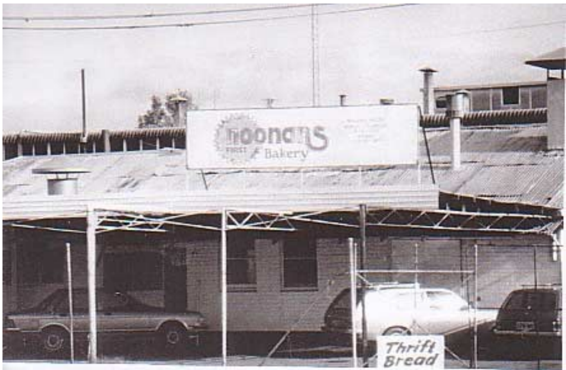
Photo 33: Noonans Bakery before demolition.
