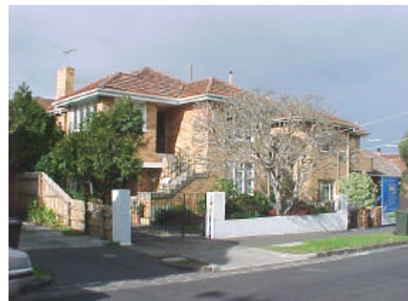
Figure 9 Double-storey flats at Nos 4 and 6
