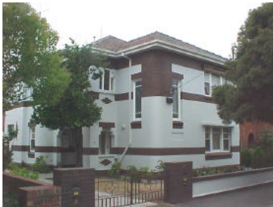
Figure 6 Moderne duplex at No 18 (1939)
