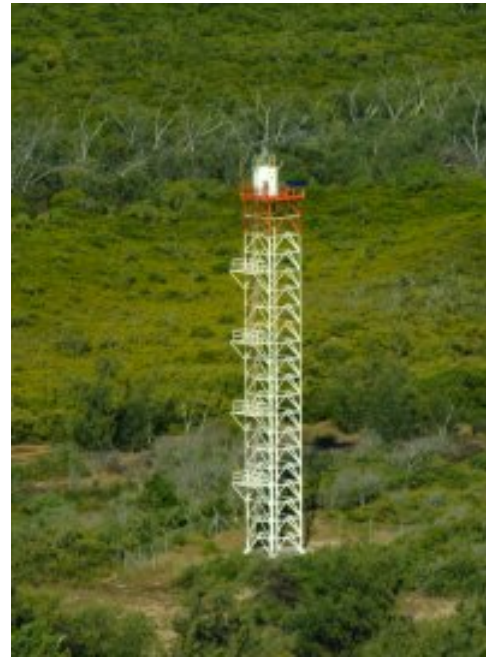
Fig 10: The new Cape Bowling Green Light house [Photograph: Winsome Bonham]
