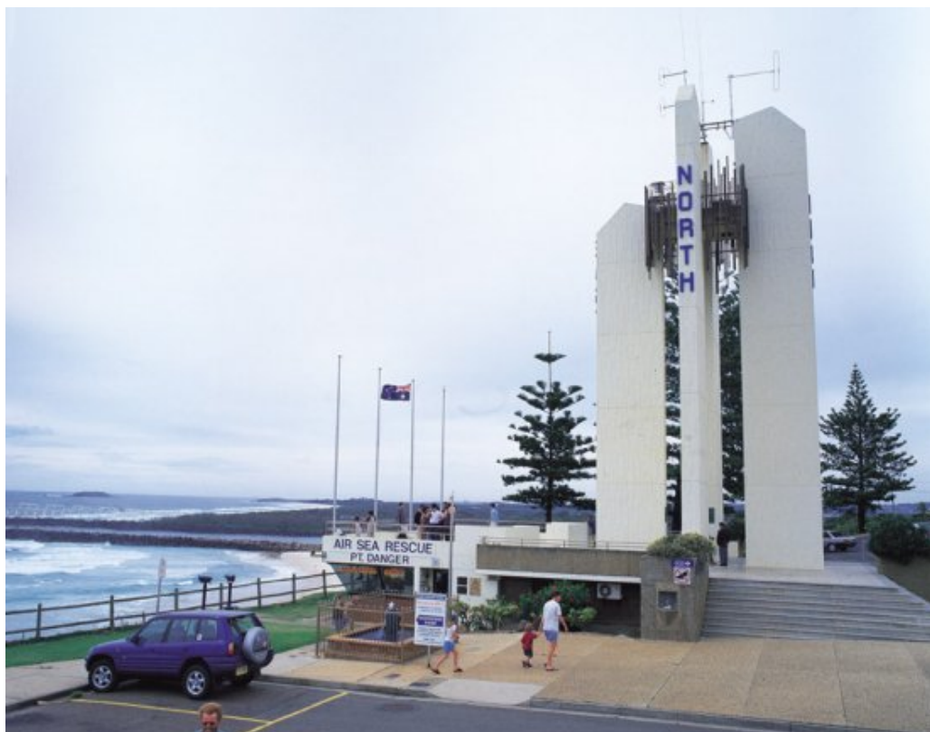
Fig 8: The Point Danger Lighthouse, noting the radial concrete blade structure typology similar to the Cleveland Point lighthouse. Photograph: Annette Flotwell
