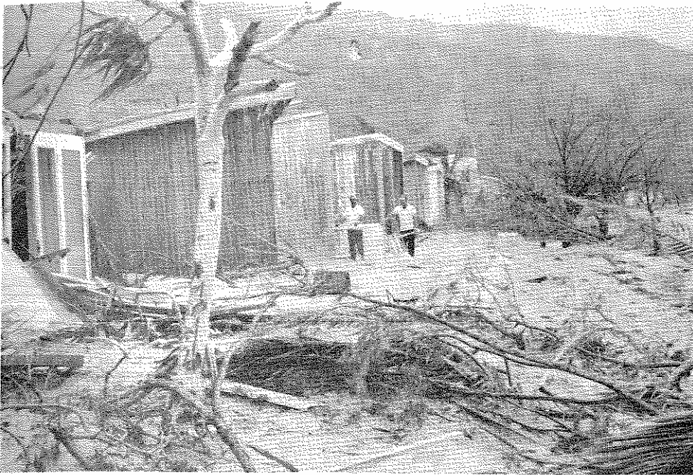
Fig. 10 Hayman Island (Note sandblasting of paintwork)
