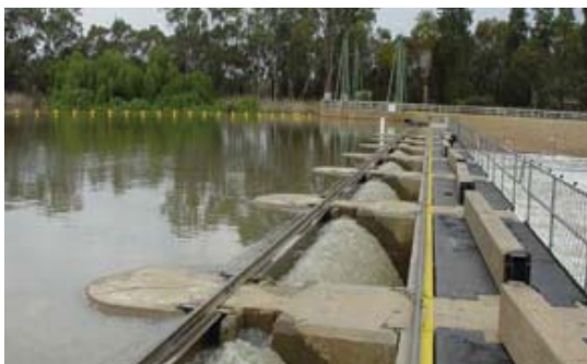
Figure 10: Lock 5 at maximum surcharge ( left ) and adjacent floodplain/wetland inundated by the weir pool raising ( right ) (Photo: Department of Water, Land and Biodiversity Conservation).
