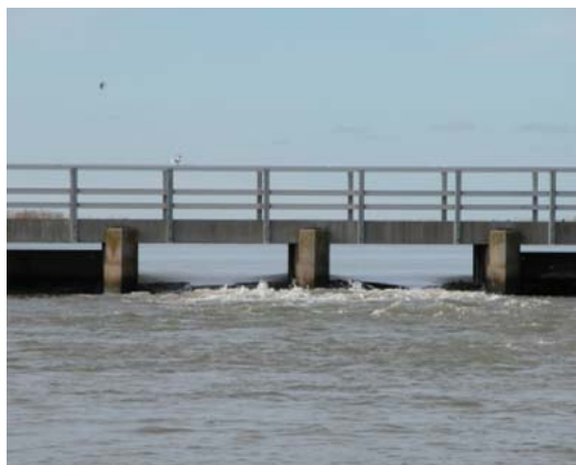
Figure 9: Two gates open at Boundary Creek Barrage (Photo: Department for Environment and Heritage).
