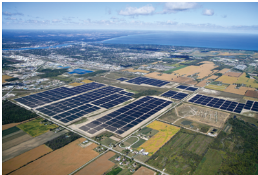
Figure 5. Canada's Sarnia Photovoltaic Power Plant became the world's largest PV plant at 80 megawatts of peak power when it was completed in September 2010. It consists of about 1.3 million thin-film PV panels covering about 966,000 square meters, but its capacity factor is expected to be only about 17 percent. (Photo courtesy of First Solar.)
