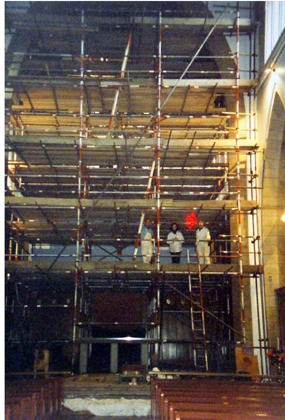
The scaffolding in the cathedral.
