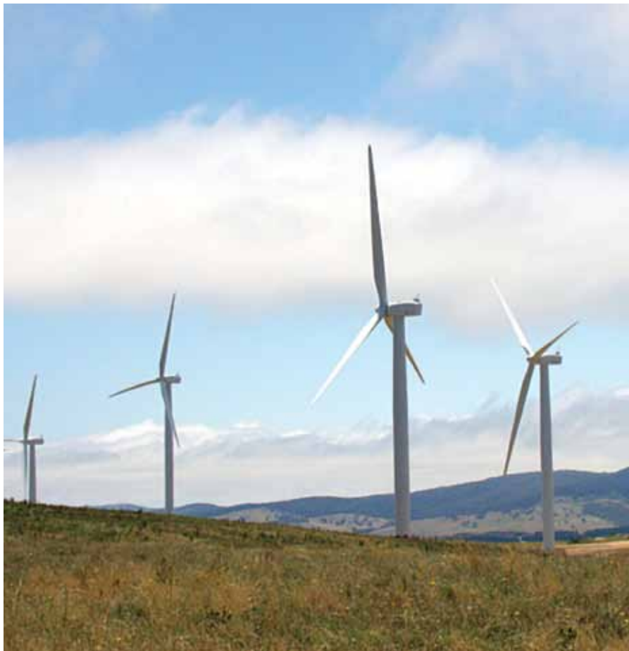
The power required to operate the desalination plant is 100 percent offset with renewable energy generated at the Capital Wind Farm near Bungendore.
