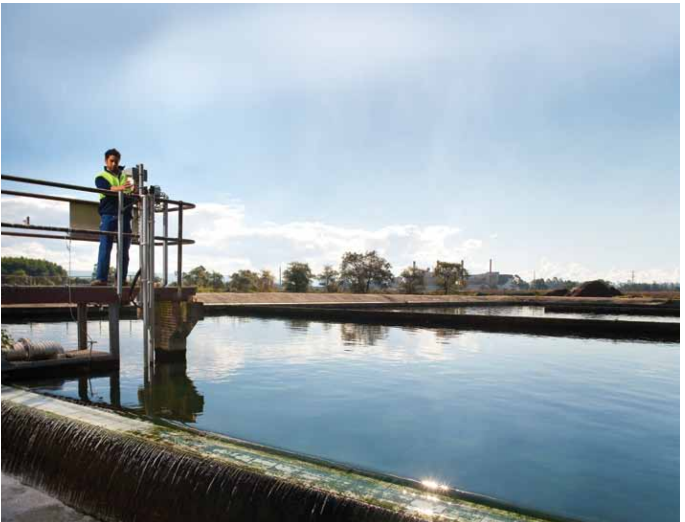
A new water recycling plant at St Marys will use the effluent from the Penrith (pictured), St Marys and Quakers Hill sewage treatment plants to provide 18 billion litres of highly treated recycled water a year to the Hawksbury-Nepean River. This will save dam water normally released to help protect the river down stream.
