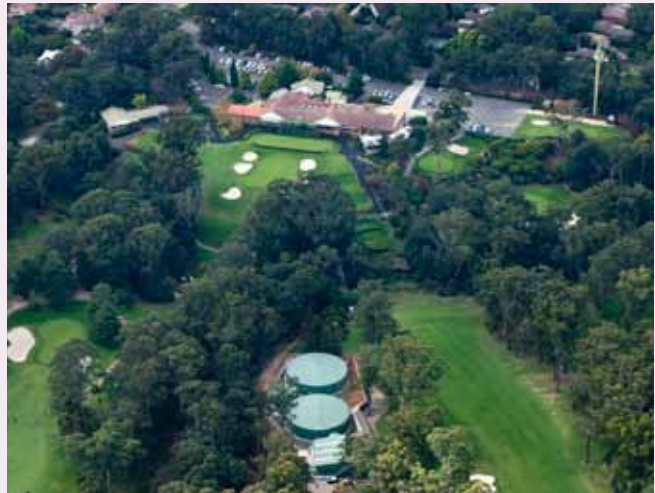
Sewer mining scheme at Pennant Hills Golf Club.
