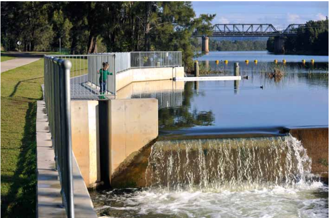
Major upgrades to a number of weirs on the Nepean River not only allow passage of new environmental flows but also help native fish move up and down the river.
