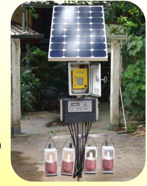
Lantern design kept simple → System's "intelligence" placed in the SCU
