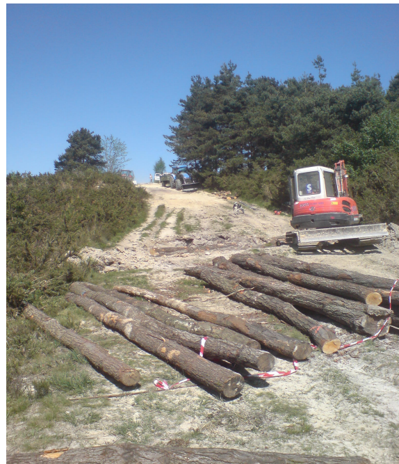
Fig. 7. Ride repairs near the Airstrip (Michael Payne).
