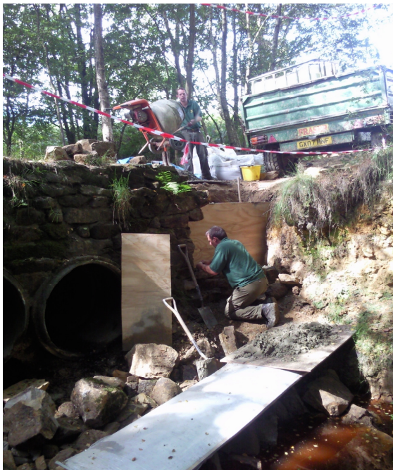
Fig. 6. Ed Burgin and Chris Sutton repairing North Pole bridge (Michael Payne).
