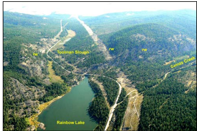
Figure 30—View east of Toolman Slough and Camas Creek rip channels converging at Rainbow Lake; rw, rip wall.
