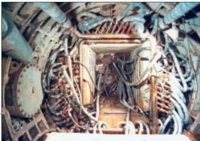
Freezer tubes in the excavation of the first shaft
