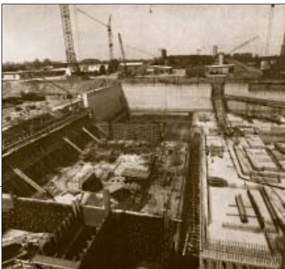
The SNR-300 in Kalkar during construction
