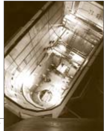
The reactor dock before the assembly of the reactor
