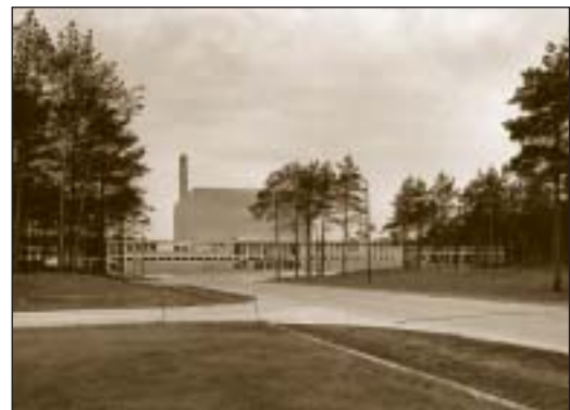
The BR1 building as completed in 1956
