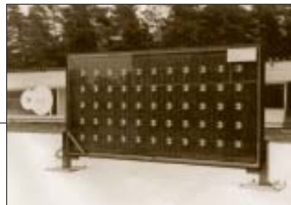
The solar collectors on the roof of the Solar Cell building
