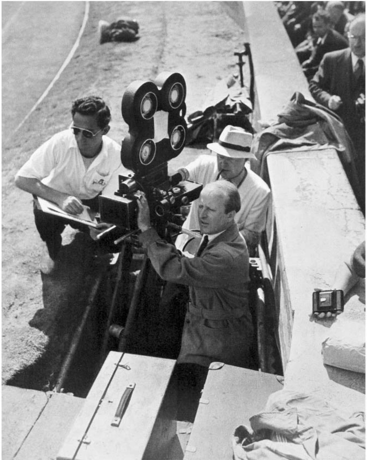
One of the pits constructed alongside the track in the Empire Stadium for filming the Olympic events. One of the camera units is at work during the course of a race.
