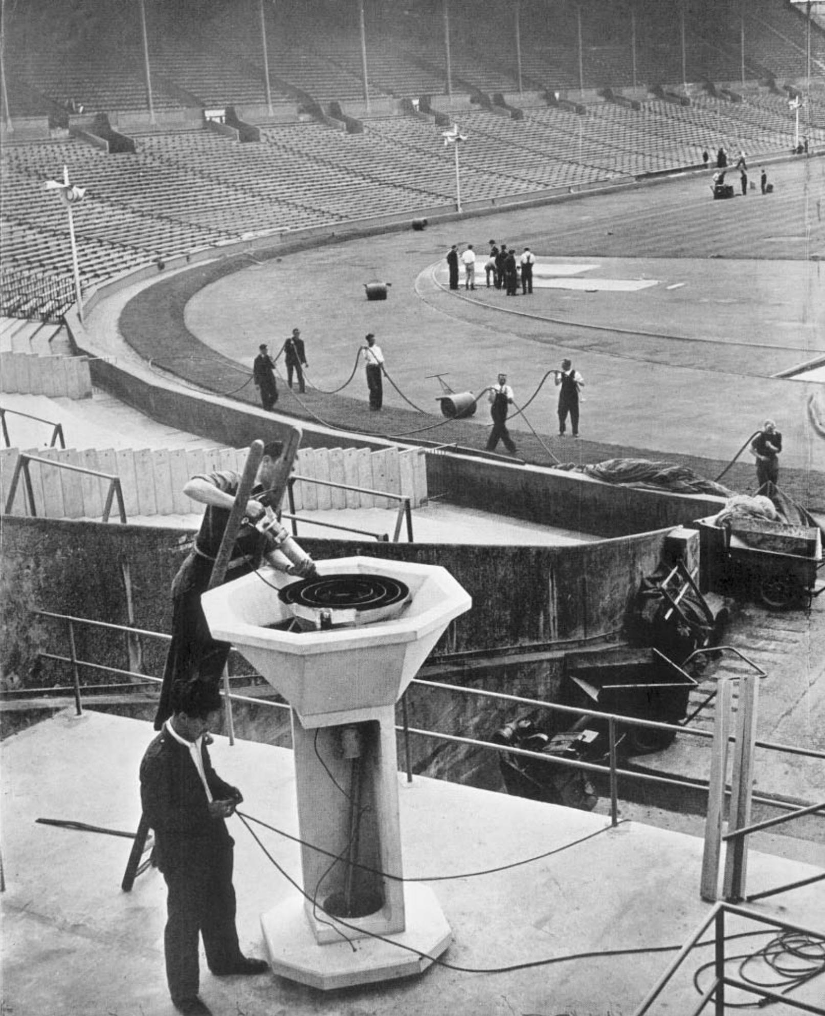
Work in progress on the preparation of the bowl for the Olympic flame at the Empire Stadium, Wembley. In the background, the finishing touches are being given to the athletic track and arena.
