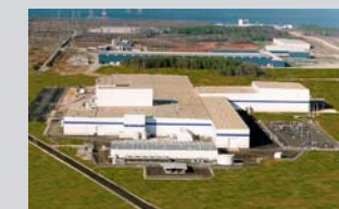
State-of-the-art lean manufacturing facility in Decatur, AL
